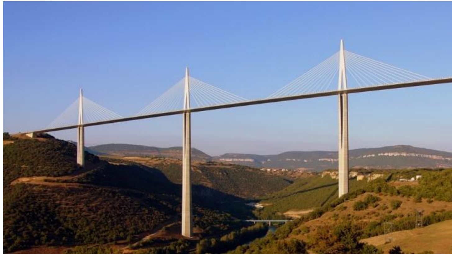
Millau Valley bridge (FR) 0.025% niobium => 60% weight reduction
