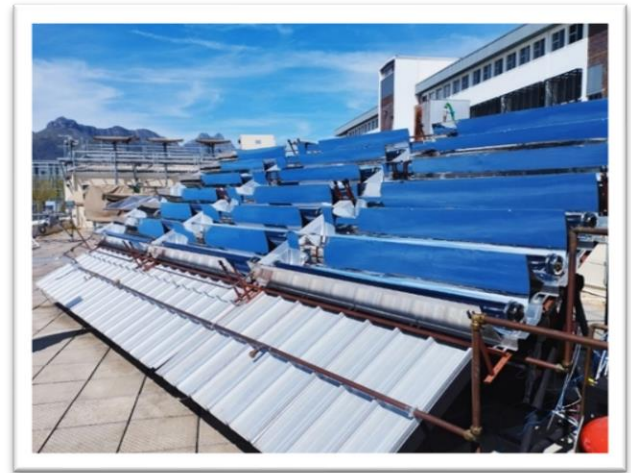
Figure 2 Solar collector array before pipe insulation
