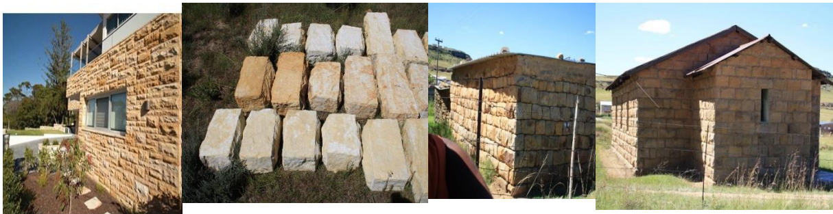
Figure 3. Sandstone used for construction. As bricks for housing in rural as well as in urban areas[18]
